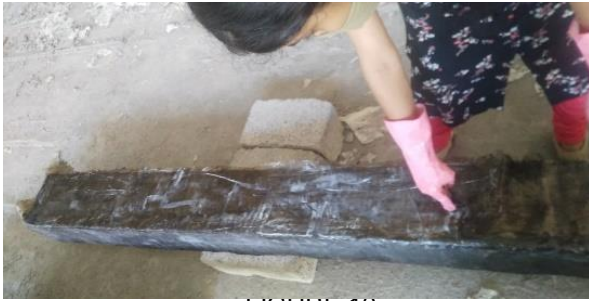
FIGURE 10 WRAPPING WITH BASALT FIBRE SHEET
