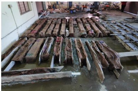
FIGURE 5 CURING OF BEAMS
