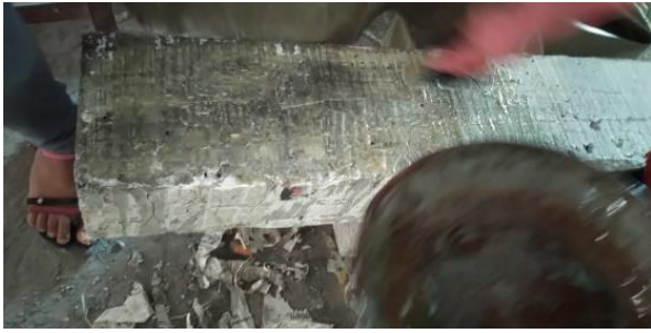
FIGURE 9 EPOXY COATING ON SURFACE OF BEAM
